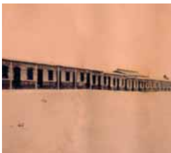
Street of the Worker's Camp, c.1930.
