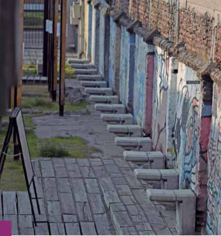
Muro interior Interior wall
